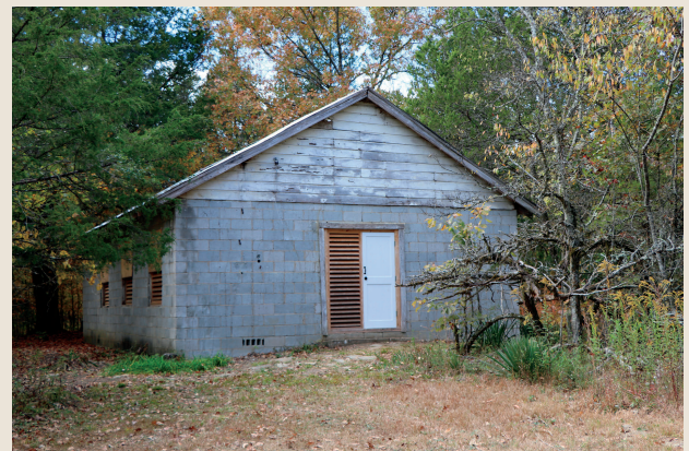
The Center Point building in October 2022, after work to repair and stabilize the building.
